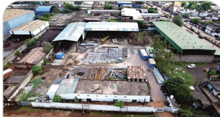
Company Aerial View
