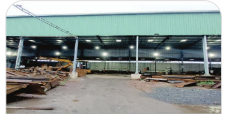
Company Shed Front view
